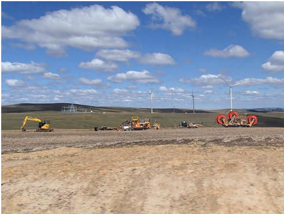
Plate 1 Cable laying equipment
